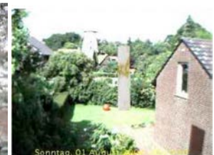
Fig.8. Column behind garage
